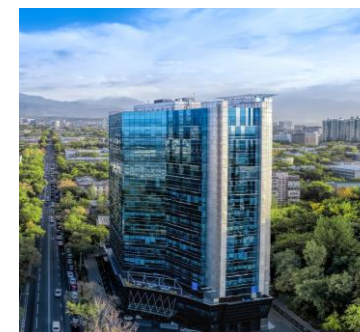
Park View Office Tower
