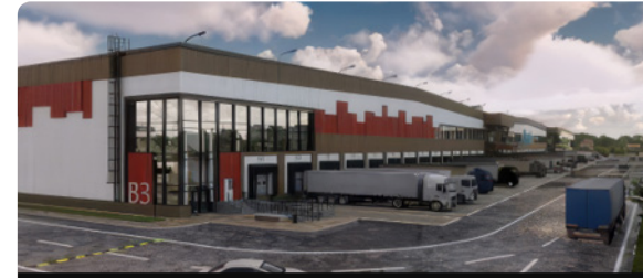
Warehouse complex, Ryazan
